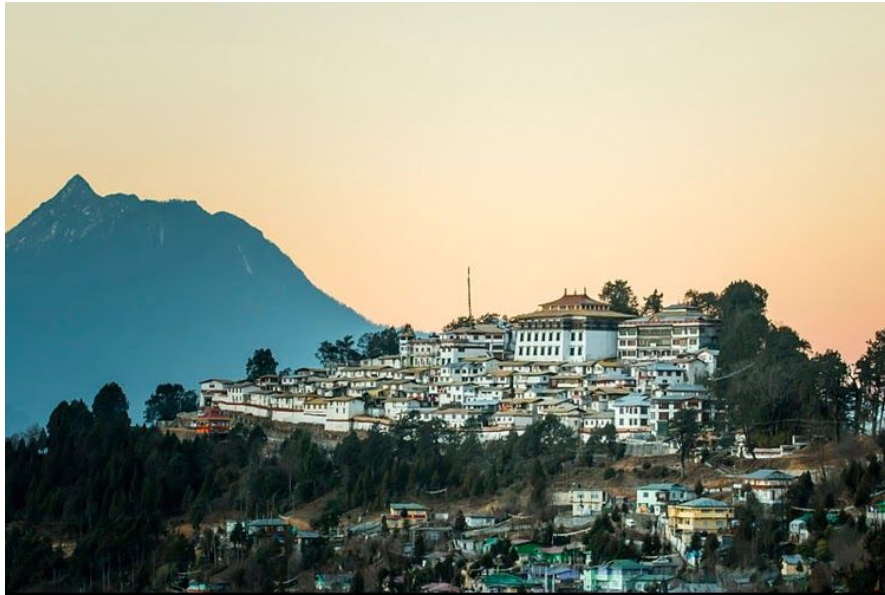
Tawang Monastery Largest Monastery in India
